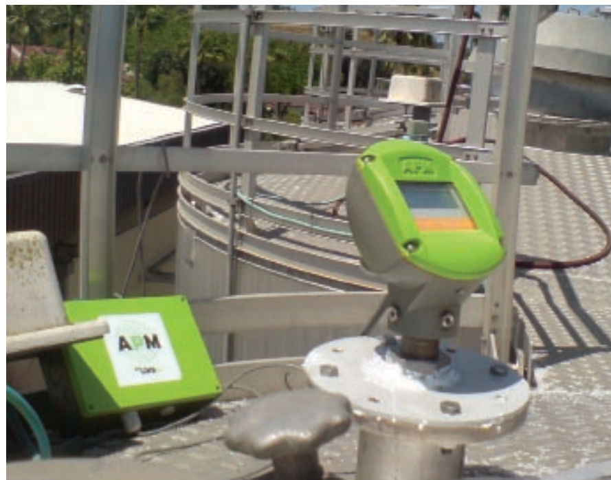
Figure 2 - Acoustic volume measurement sensor measuring PE pellets (photo courtesy APM Automation Solutions Ltd)
